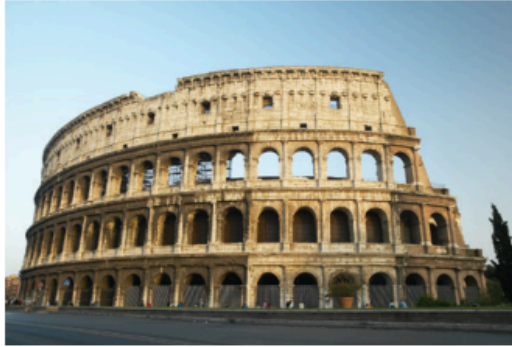
Figure 13.2 ■ The Roman Coliseum, showing the use of multiple arches. Image © 2006 Jupiter Images Corporation.
