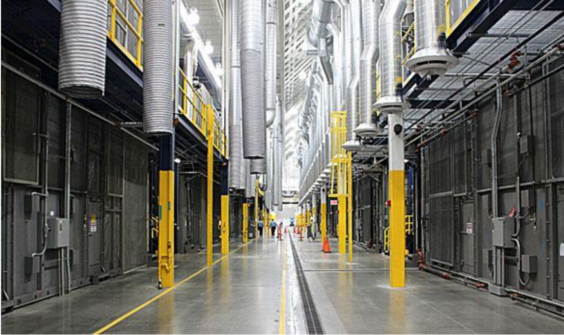
Figure 27 Photo of the ovens of two carbon fiber lines
