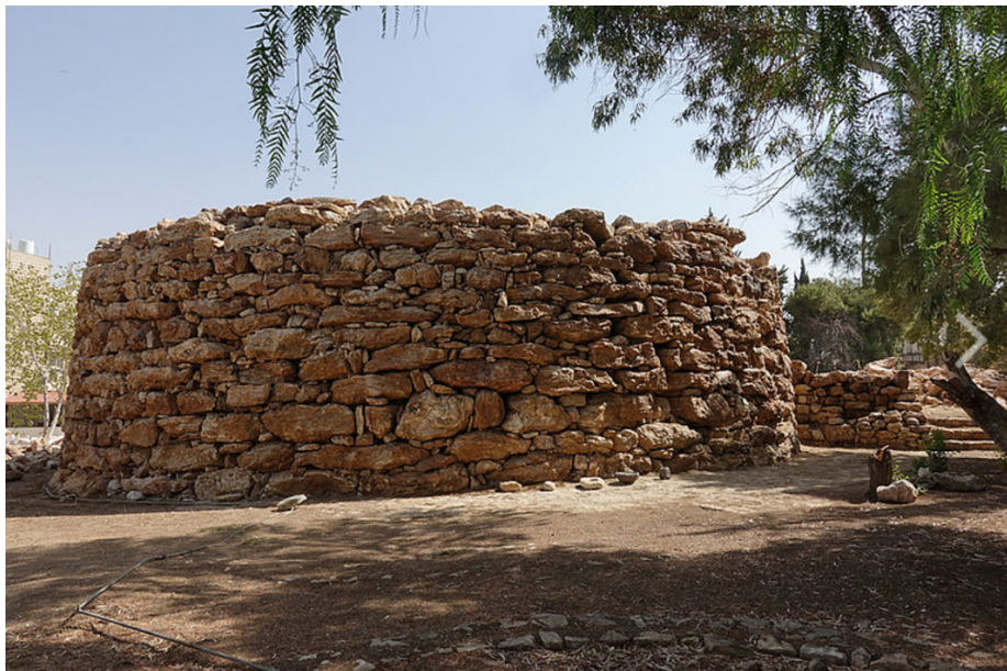
Figure 27: Ammonite tower outside Amman ( https://universes.art/en/art-destinations/jordan/amman/museums/ammonite-watchtower )
